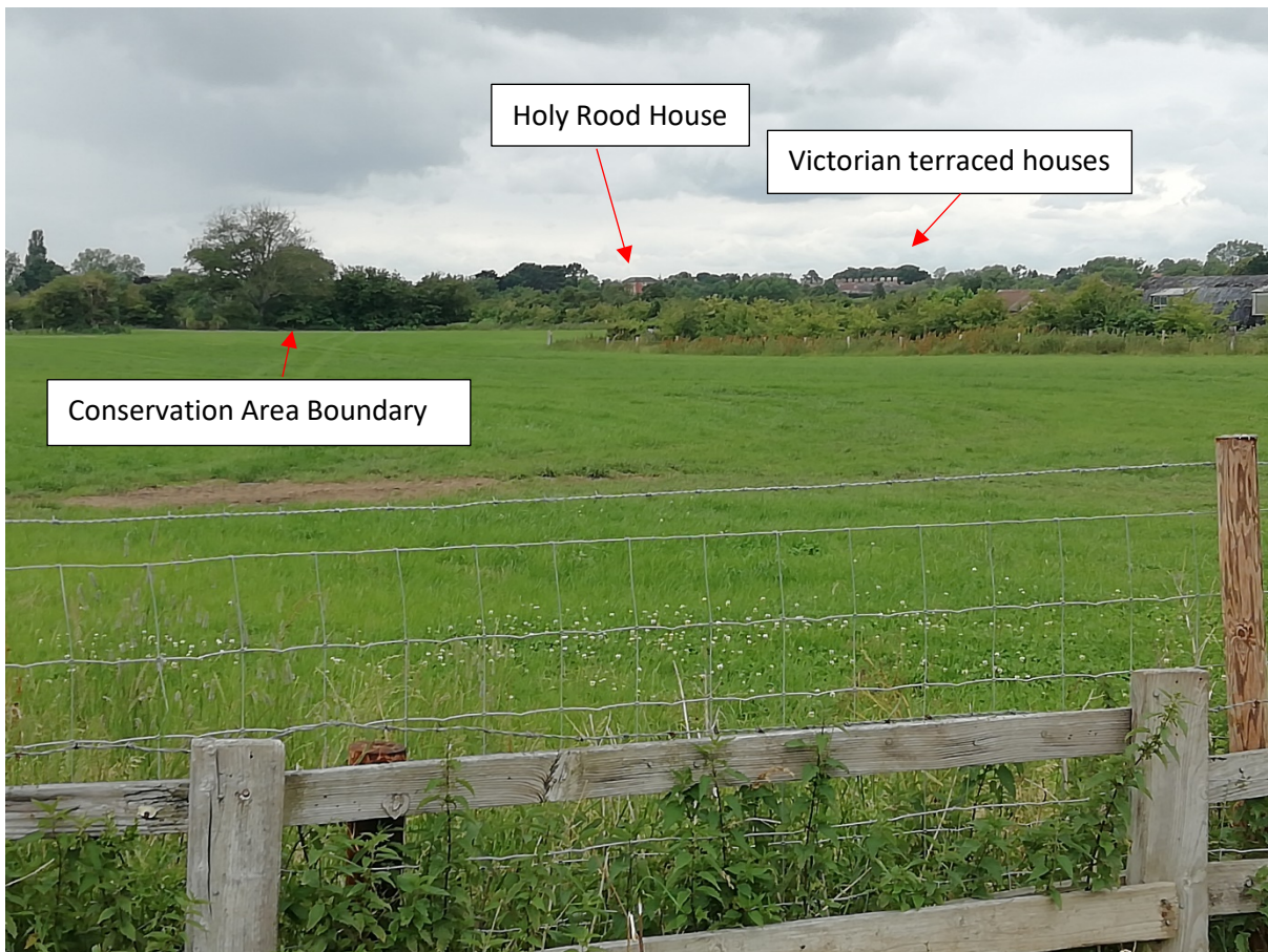
Fig 1 Across application site to historic buildings within Conservation Area (boundary is tree line)
