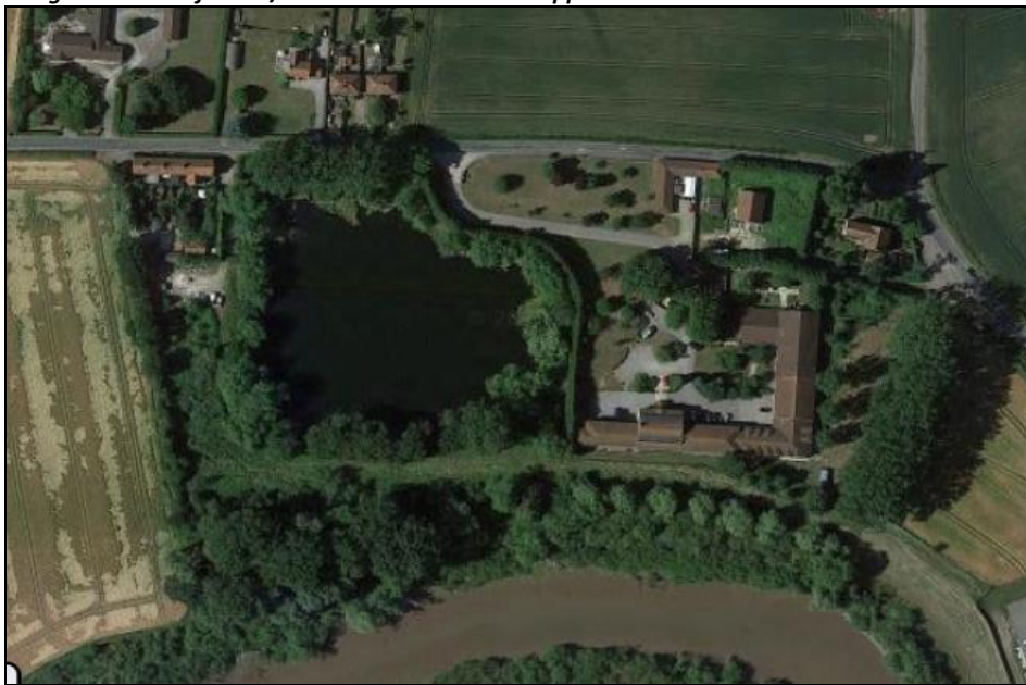
Image 1: extent of shrub/tree-cover to be lost on application site
